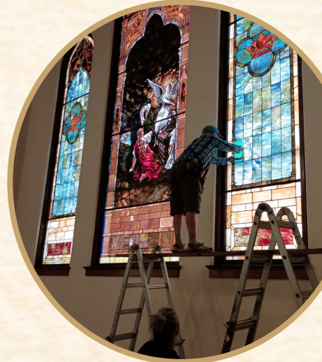
Interior Stain Glass Restoration
