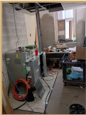
Old and New Elevator Panels
